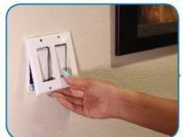
Remove visible screws and take off the switch plate.
