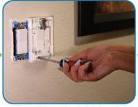
Add Ecolink mechanical light switch over the light switch and replace screws removed.
